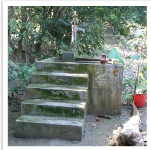
16 Raised Platform Tube Well
